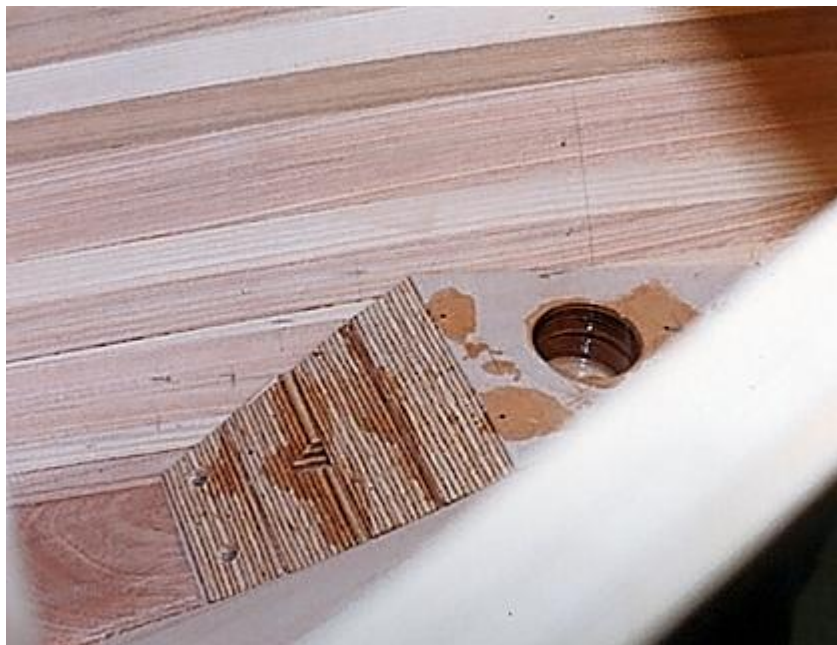
Mast step with drainage hole
